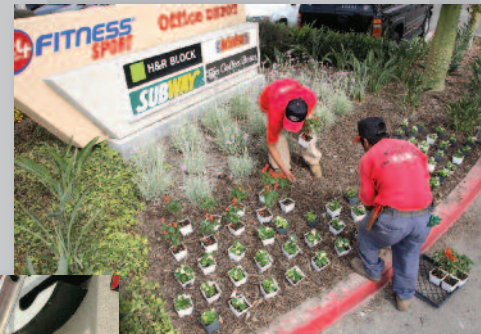
Landscape Renewal and Irrigation Installation
