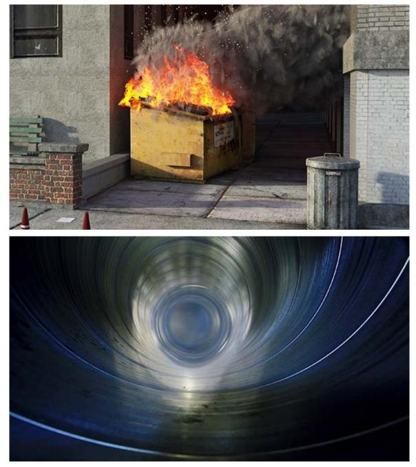
Chutes are either rectangular or round. The shape may be determined by construction constraints or the manufacturer's equipment. However, when presented with the option, one should consider the benefits of a round trash chute. Much like the infamous query "Why are manhole covers round?" – a round chute is more likely to prevent oversized items from becoming wedged as they cannot be rotated for a different fit as rectangular chutes allow.
