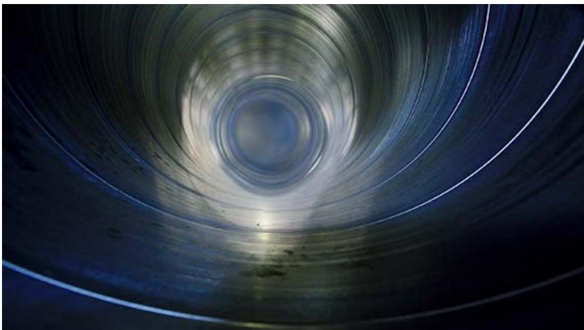
Chutes are either rectangular or round. The shape may be determined by construction constraints or the manufacturer's equipment. However, when presented with the option, one should consider the benefits of a round trash chute. Much like the infamous query "Why are manhole covers round?" - a round chute is more likely to prevent oversized items from becoming wedged as they cannot be rotated for a different fit as rectangular chutes allow.
