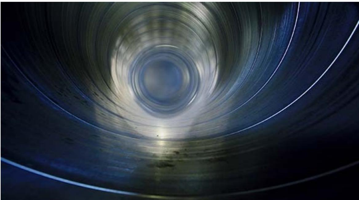
Chutes are either rectangular or round. The shape may be determined by construction constraints or the manufacturer's equipment. However, when presented with the option, one should consider the benefits of a round trash chute. Much like the infamous query "Why are manhole covers round?" - a round chute is more likely to prevent oversized items from becoming wedged as they cannot be rotated for a different fit as rectangular chutes allow.
